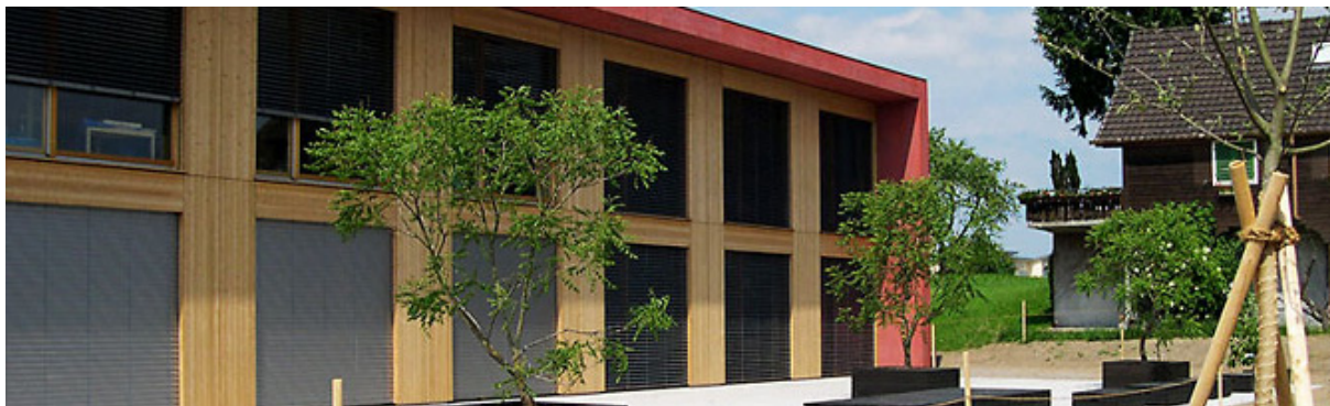
Fassade in Thermowood
